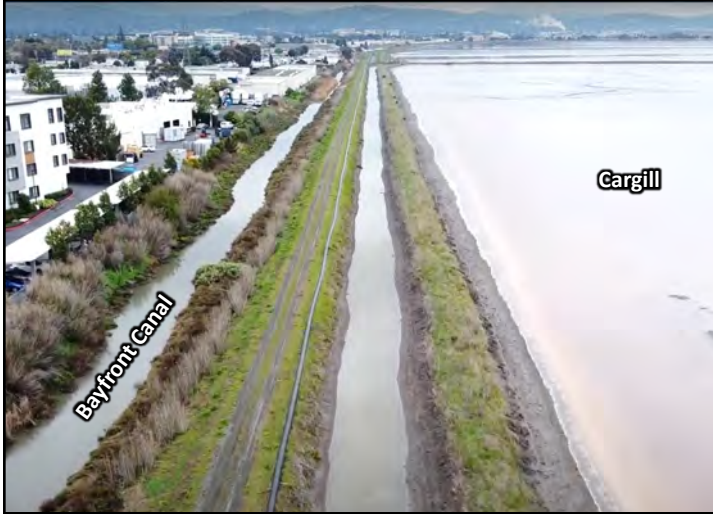
From Marsh Road towards Seaport Boulevard
