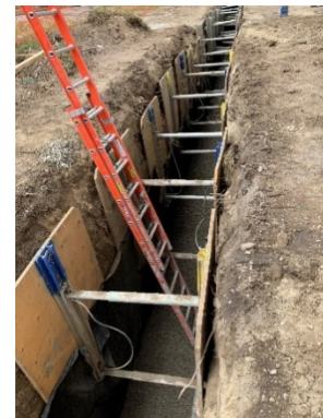
Figure 3. Diversion Pipe Trench with Shoring
