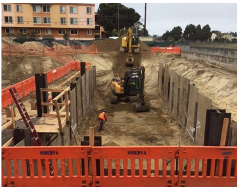
Figure 1. Excavation for the Grit Chamber Structure
