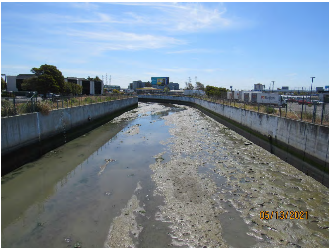
Photos 20 & 21 – Top photo shows Colma Creek looking upstream from the Produce Avenue bridge. Sediment accumulated near the northern (right) bank is to be dredged during the 2021 maintenance season. Bottom photo shows Colma Creek looking downstream from the San Mateo Avenue Bridge.
