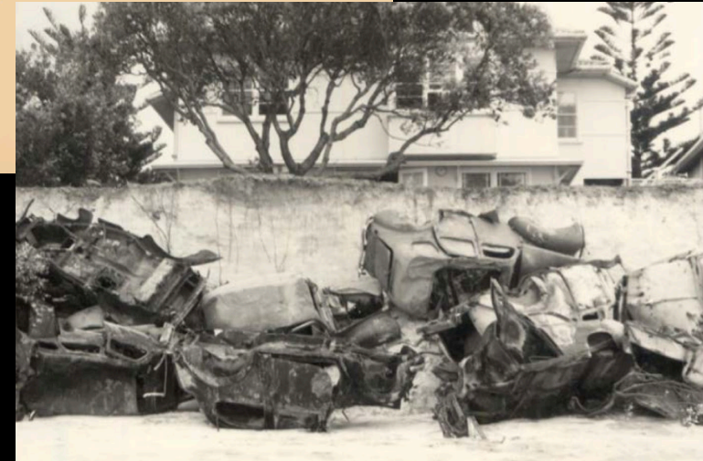
Figure 5 Use of car bodies to protect against storm erosion in 1967 (Source: GCCC)
