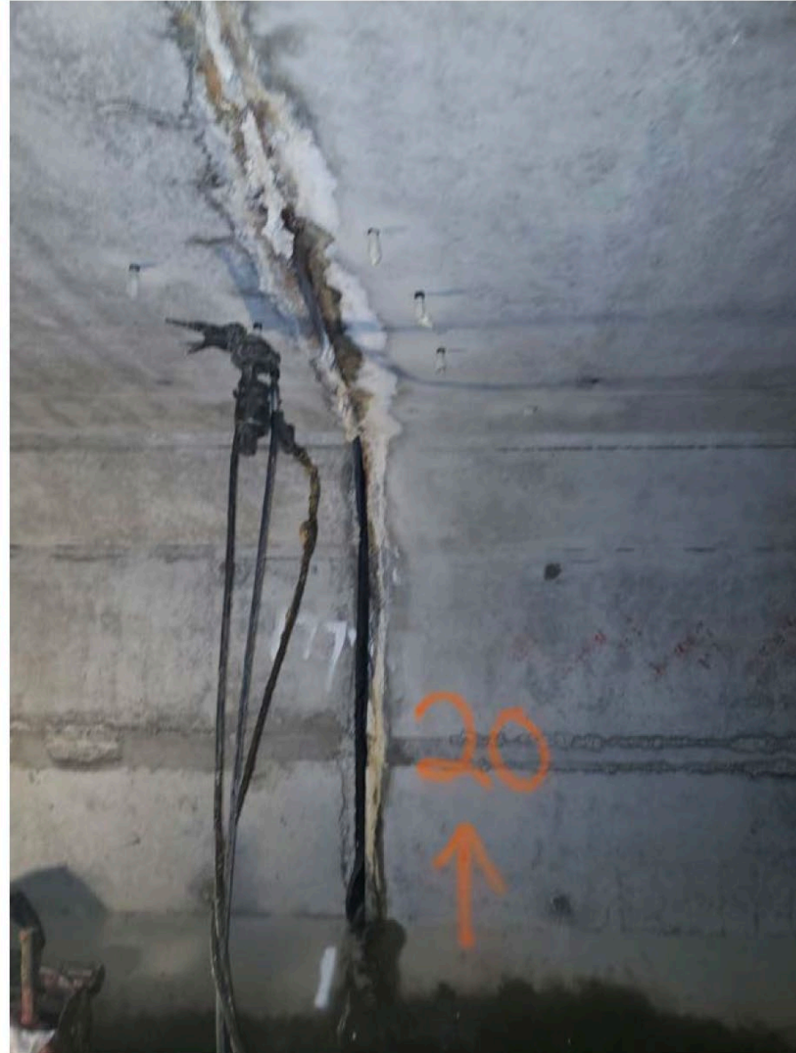
Photos 3 & 4 – El Camino Real box culvert repairs in progress. Left photo shows holes for the polymer injection were being drilled. Right photo shows polymer material being injected into the holes which is engineered to expand and fill cracks and voids in the concrete.
