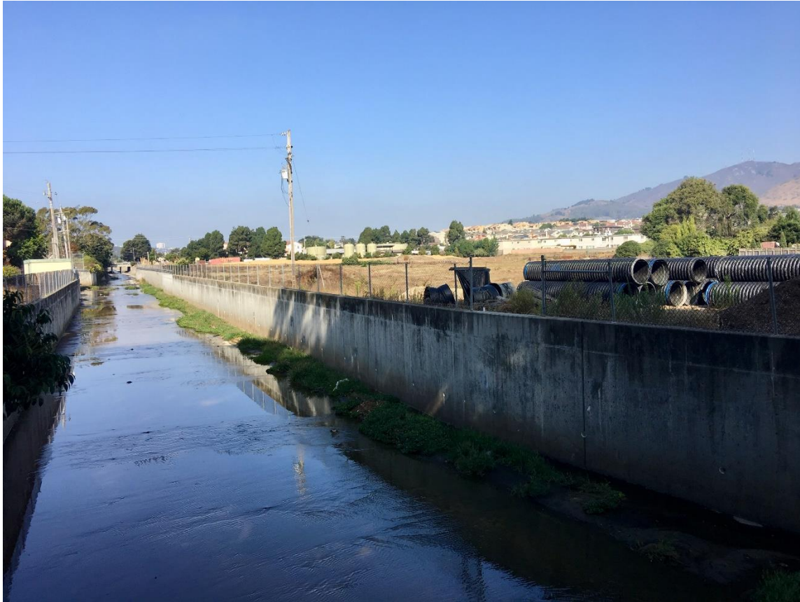
Upstream View at 1 st Pedestrian Bridge
