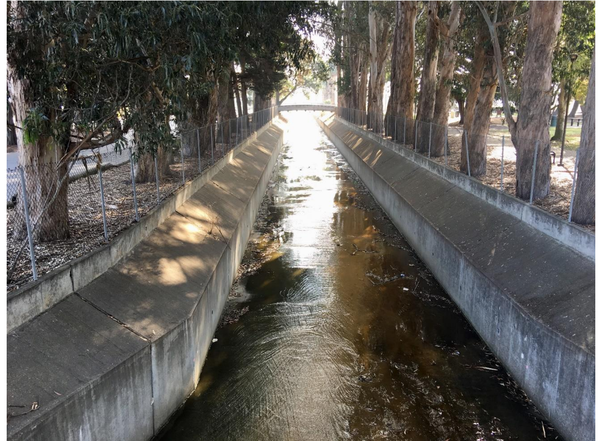
Downstream View at 1 st Pedestrian Bridge
