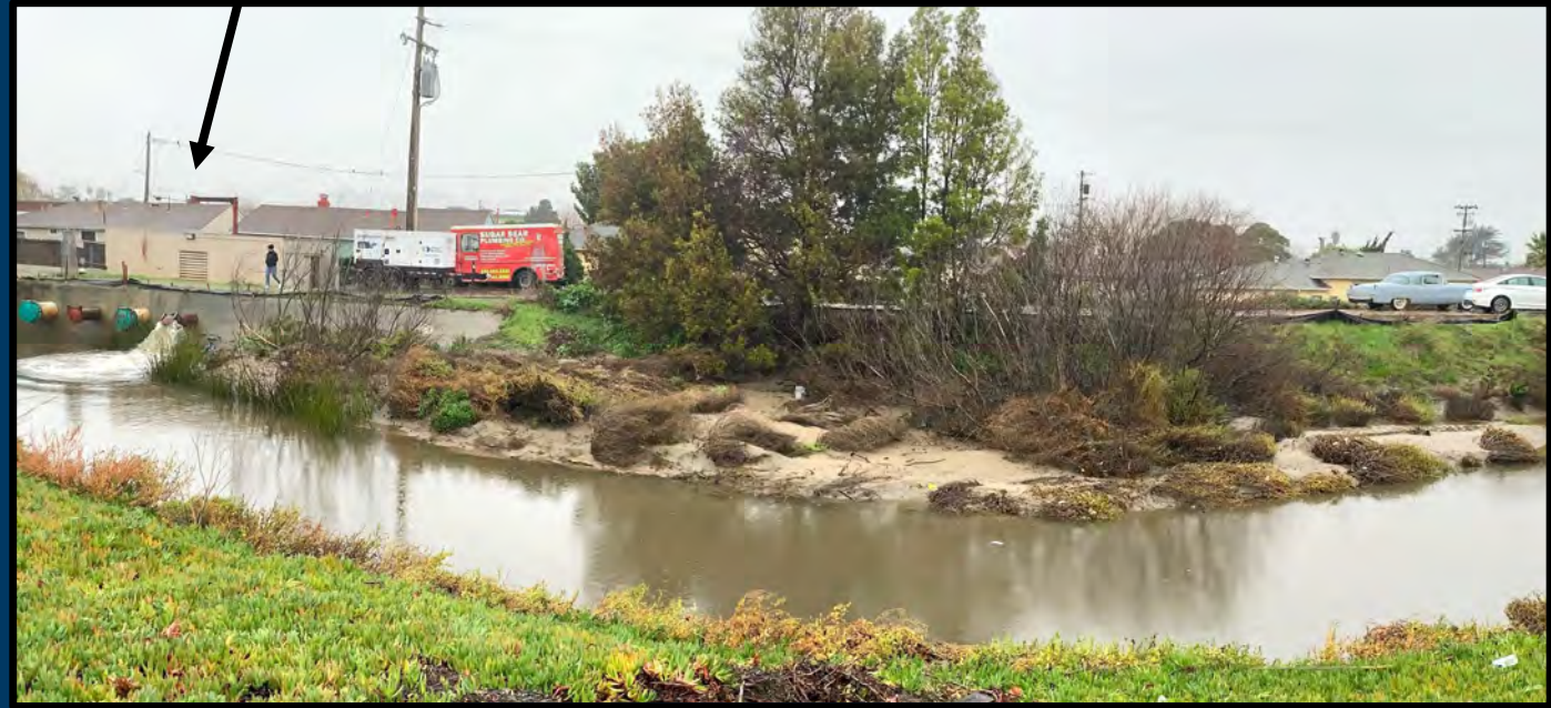
Walnut St. Pump Station
