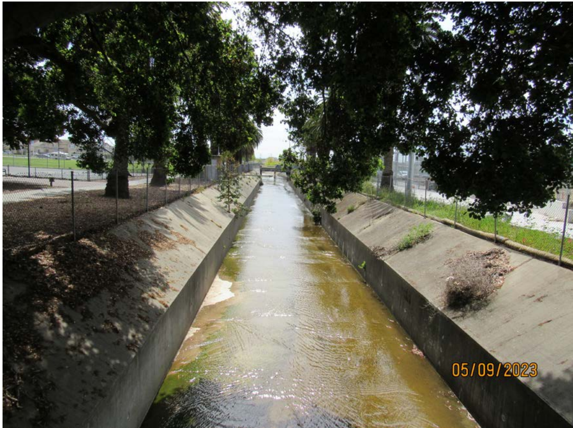
Photos 27 & 28 – Top photo shows Colma Creek looking upstream from Orange Avenue bridge. Bottom photo shows Colma Creek looking downstream from the Orange Park pedestrian bridge. Overgrown vegetation observed in the wall joints between the Orange Avenue bridge and Orange Park pedestrian bridge.
