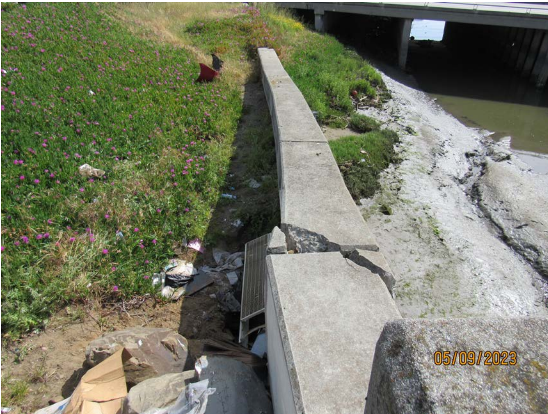
Photos 15 & 16 – Top photo shows crack in channel wall downstream of Produce Avenue bridge. Bottom photo shows sinkhole forming behind the wall filled with dumped debris. OneShoreline and SSF staff are aware of the conditions of the channel wall and sinkhole.
