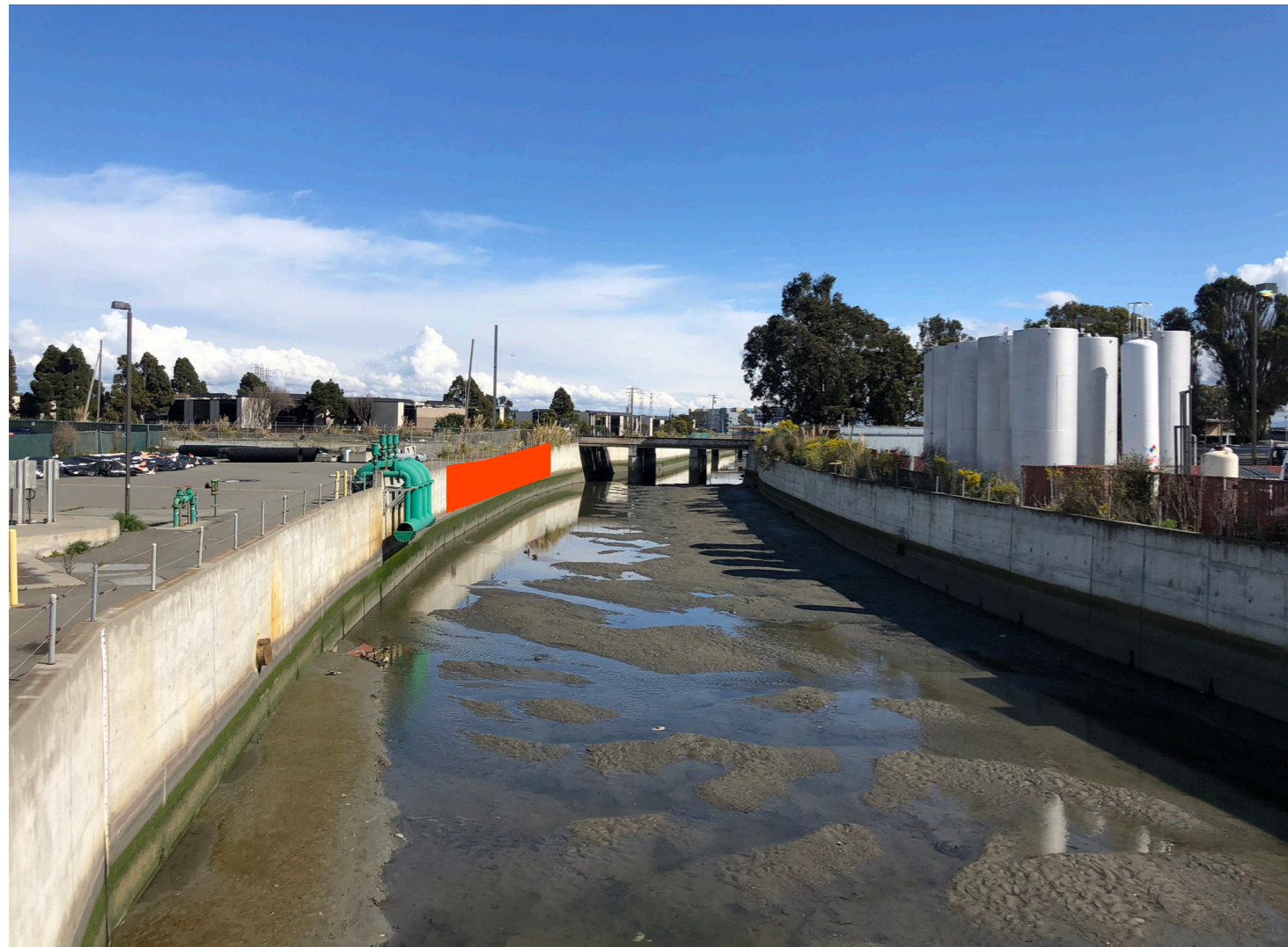
Partial removal of existing flood wall
