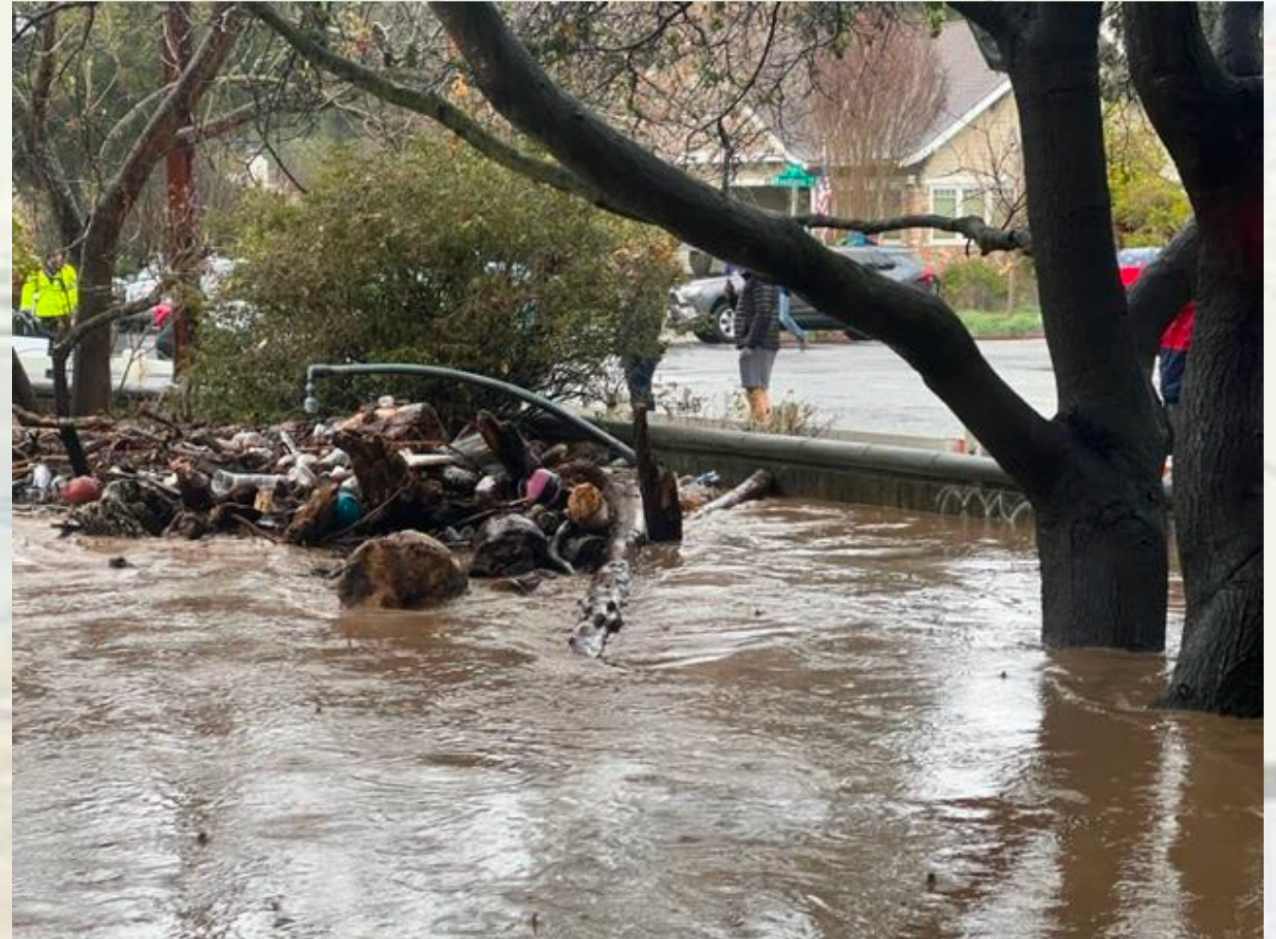
Photo credit: P. Burt, 31 Dec. 2022. Upstream face of Pope-Chaucer bridge
