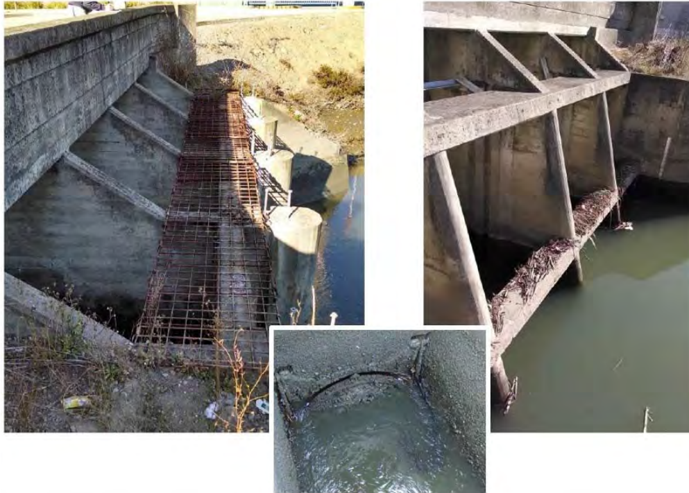
Downstream (Left), Upstream (Right) & Flapgate (Middle)
