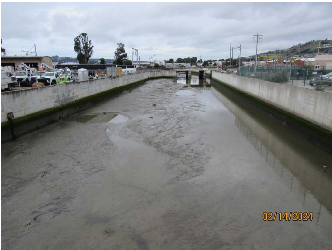
Photos 13 & 14 – Top photo shows Colma Creek looking downstream from the San Mateo Avenue bridge . Bottom photo shows Colma Creek looking upstream from the San Mateo Avenue bridge.
