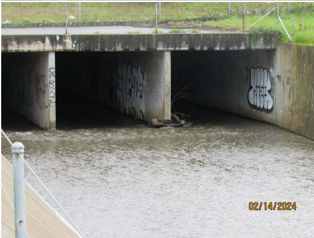
Photos 27 & 28 – Top photo shows Colma Creek looking downstream from the SSF BART Station culvert. Bottom photo shows minor debris at the inlet to the SSF BART Station box culvert at McLellan Drive. Note the water level in the channel at this point in the day increased following rain event. County recommends OneShoreline to coordinate with SSF staff to remove the debris per the MOA between OneShoreline and SSF.
