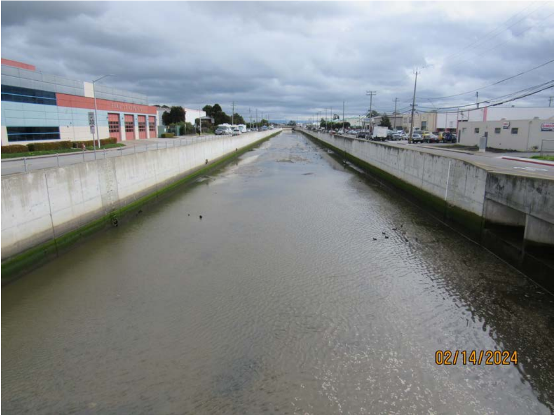
Photos 17 & 18 – Top photo shows Colma Creek looking upstream from Spruce Avenue bridge. Bottom photo shows Colma Creek looking downstream from Spruce Avenue bridge.
