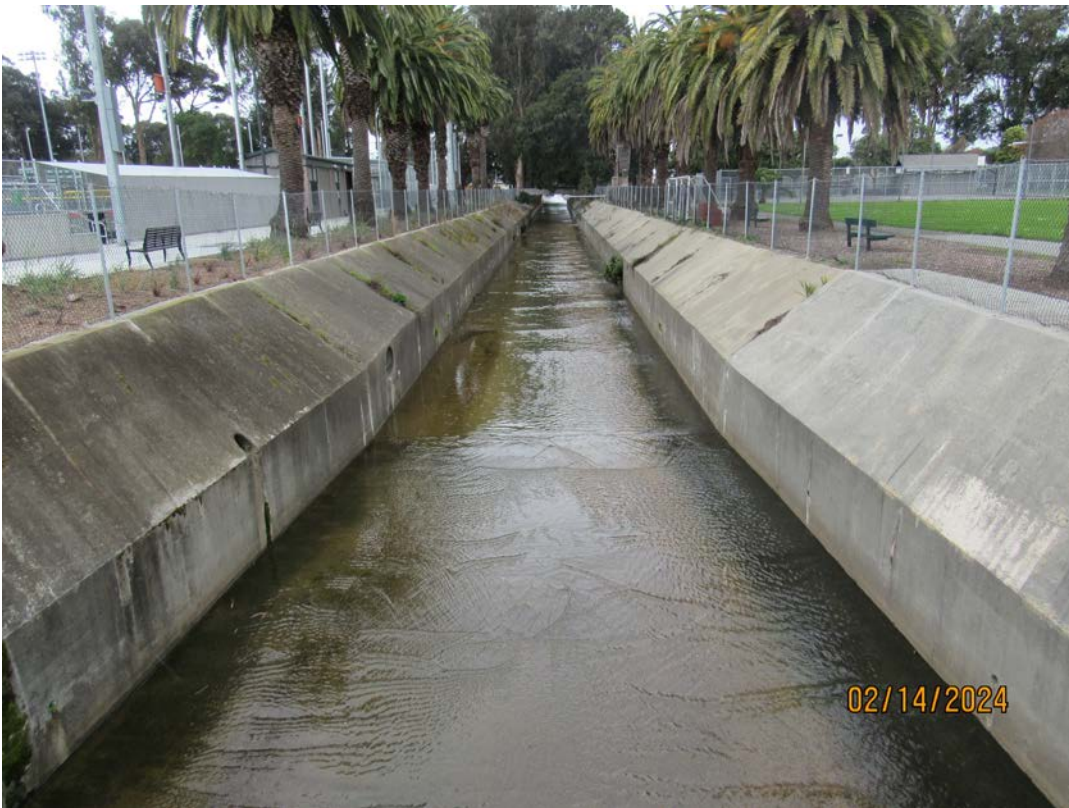
Photos 21 & 22 —Top photo shows Colma Creek looking downstream from the Orange Avenue bridge. Bottom photo shows Colma Creek looking upstream from Orange Avenue bridge.
