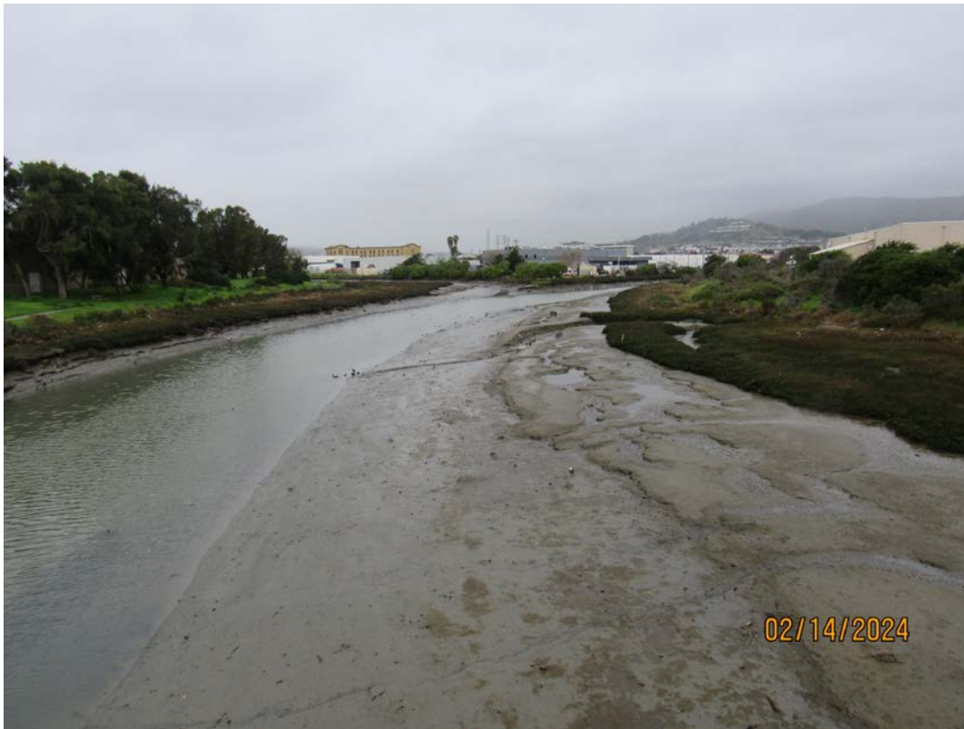
Photos 1 & 2 – Top photo shows Colma Creek looking downstream from the Bay Trail pedestrian bridge. Bottom photo shows Colma Creek looking upstream from the pedestrian bridge.
