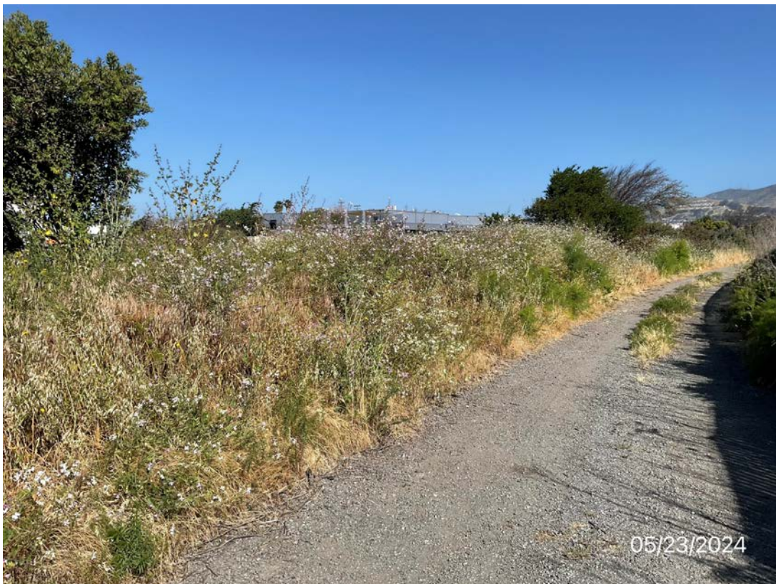
Photos 3 & 4 – Top and bottom photos show previous homeless encampments sites between the Bay Trail pedestrian bridge and Utah Avenue cleared of encampments. However, some trash and debris still remain. Cable fence not adequately repaired. OneShoreline and County planning on clearing trash/debris in these areas and maintain/replace native vegetation during future cleanup/planting events.
