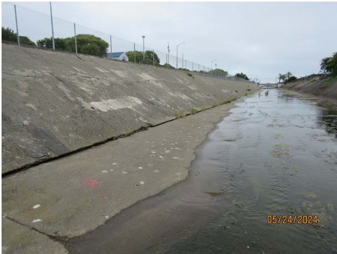
Photos 21 & 22 – Top photo shows minor debris accumulated at the dissipator teeth upstream of the Spruce Avenue bridge.. Bottom photo shows trapezoidal wall separation at channel floor developing upstream of the Spruce Avenue bridge. Consultant firm has assessed the conditions of the concrete channel and recommends a geotechnical investigation be conducted to identify causes for the soil settlement. County will monitor the separation in future inspections.
