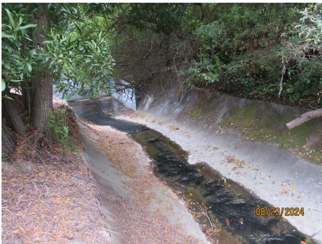
Photos 37 & 38 – Top photo shows old Colma Creek channel downstream of the El Camino Real bridge at the Mission Road intersection. Bottom photo shows Colma Creek channel facing downstream looking at the diversion structure and junction with the Old Channel.
