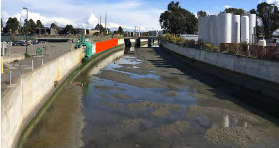
Partial removal of existing flood wall
