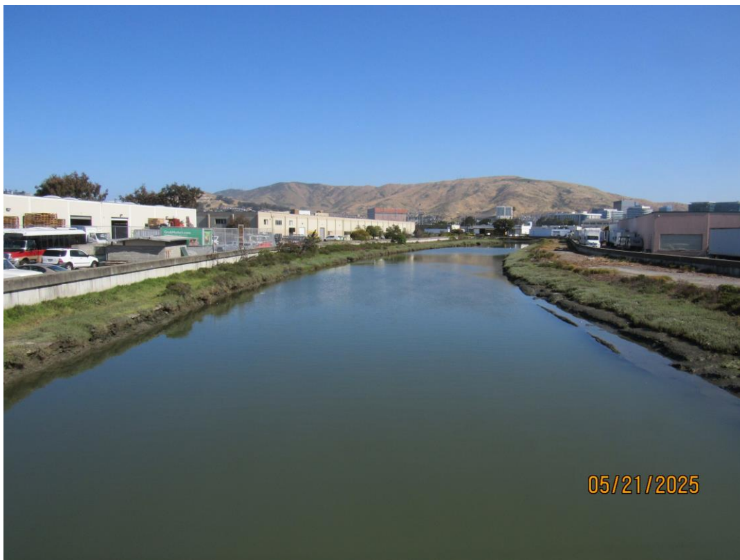
Photos 5 & 6 – Top photo shows Colma Creek looking downstream from the Utah Avenue bridge. Bottom photo shows Colma Creek looking upstream from Utah Avenue.
