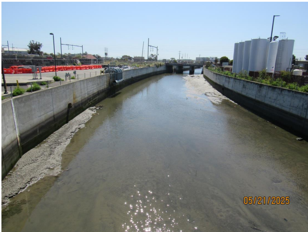
Photos 17 & 18 – Top photo shows Colma Creek looking upstream from Linden Avenue bridge. Bottom photo shows Colma Creek looking downstream from the Linden Avenue bridge.
