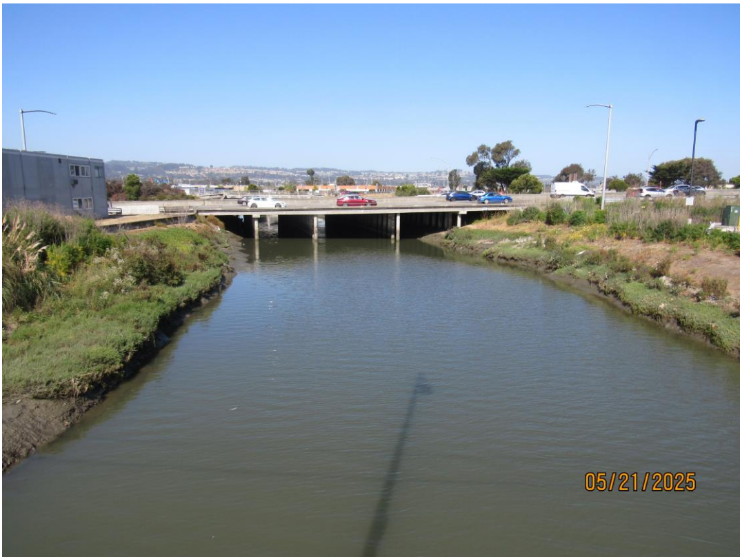
Photos 9 & 10 – Top photo shows Colma Creek looking downstream from the S. Airport Blvd. bridge. Bottom photo shows Colma Creek looking upstream from S. Airport Blvd. facing the Hwy 101 crossing. Trash from various sources including storm drains and illegal dumping continues to be an issue. A potential encampment was observed under S. Airport Blvd..
