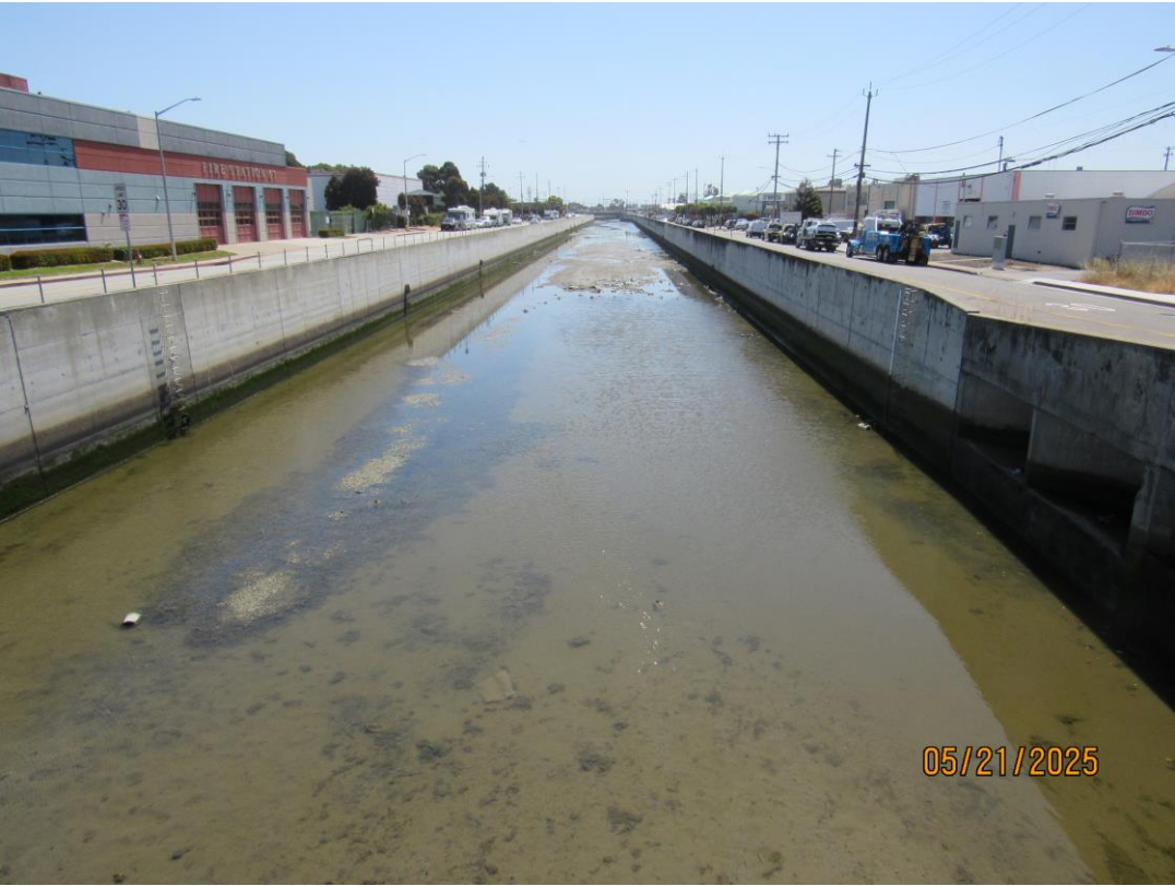
Photos 19 & 20 – Top photo shows Colma Creek looking upstream from Spruce Avenue bridge. Bottom photo shows Colma Creek looking downstream from Spruce Avenue bridge.
