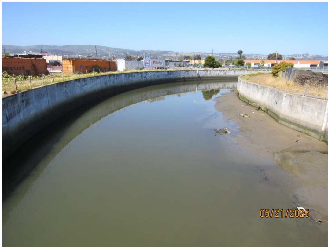
Photos 11 & 12 – Top photo shows Colma Creek looking downstream from the Produce Avenue bridge facing the Hwy 101 crossing. Bottom photo shows Colma Creek looking upstream from the Produce Avenue bridge.
