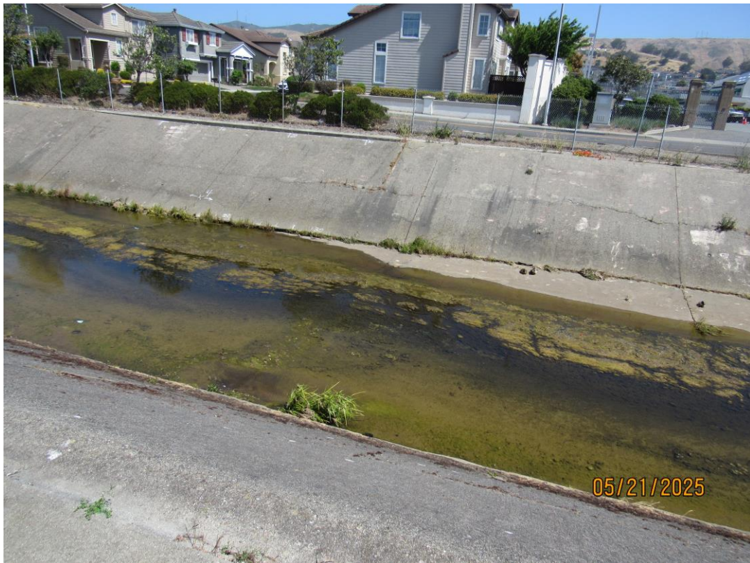
Photos 21 & 22 – Top photo shows minor debris accumulated at the dissipator teeth upstream of the Spruce Avenue bridge. Bottom photo shows trapezoidal wall separation at channel floor developing upstream of the Spruce Avenue bridge. This section was included in a geotechnical investigation to identify causes for the soil settlement. County recommends OneShoreline to continue monitoring the separation in future inspections.
