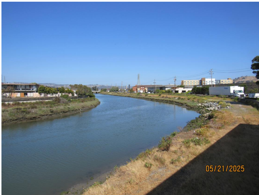
Photos 7 & 8 – Top photo shows Colma Creek looking downstream towards the Utah Avenue bridge. Bottom photo shows Colma Creek looking upstream towards the S. Airport Blvd. bridge. Trash from various sources including storm drains and illegal dumping continues to be an issue.
