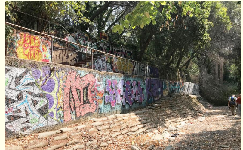
Concrete terrace at Site 2
