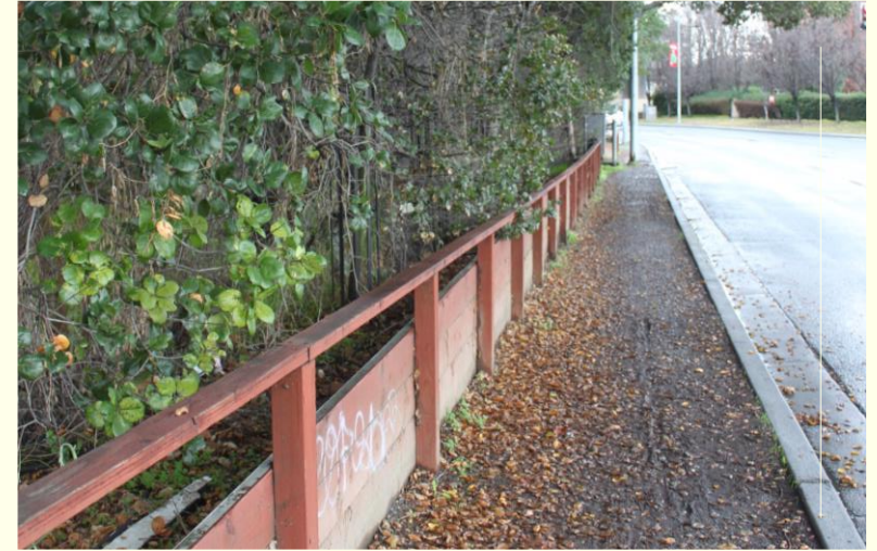
Temporary wooden parapet at University Ave
