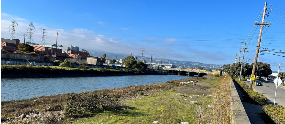
Figure 4. Downstream of Airport Boulevard along Mitchell Avenue, soft-bottom tidal reach
