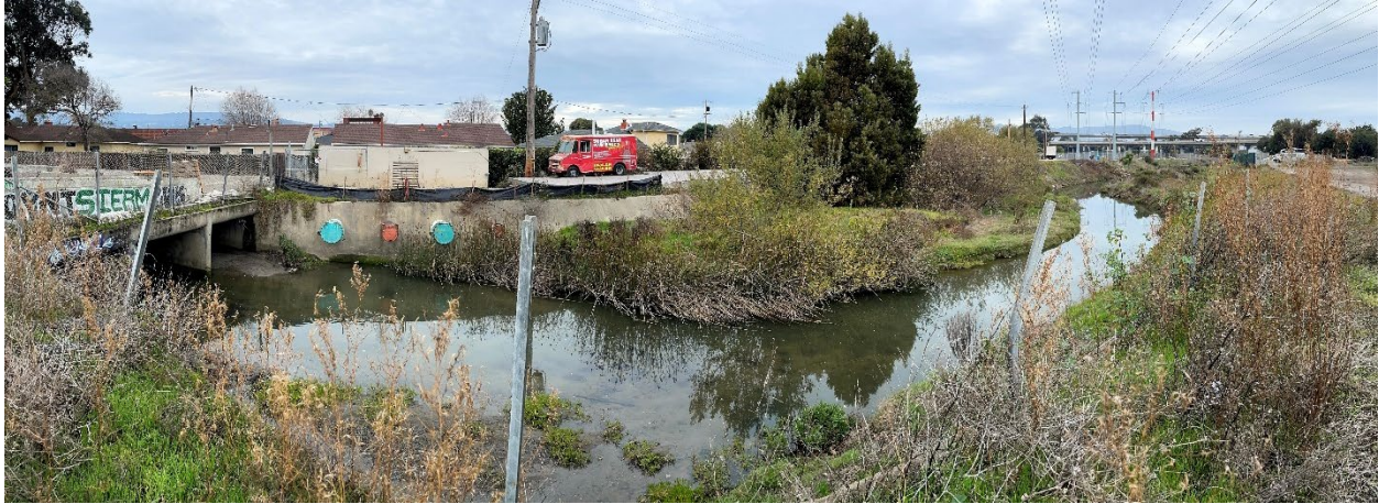
Figure 7. North Channel at Walnut Pump Station
