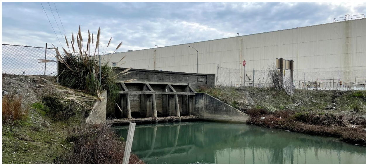
Figure 6. San Bruno Creek Tide Gate at North Access Road
