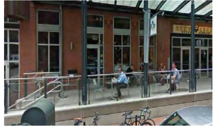
Flood-Proofed Building, Boston Waterfront
