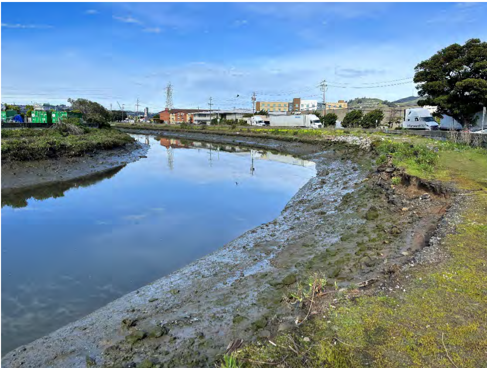
Photos 9 & 10 — Top photo shows Colma Creek looking downstream towards the Utah Avenue Bridge. Bottom photo shows Colma Creek looking upstream towards the S Airport Blvd Bridge. Low tide.
