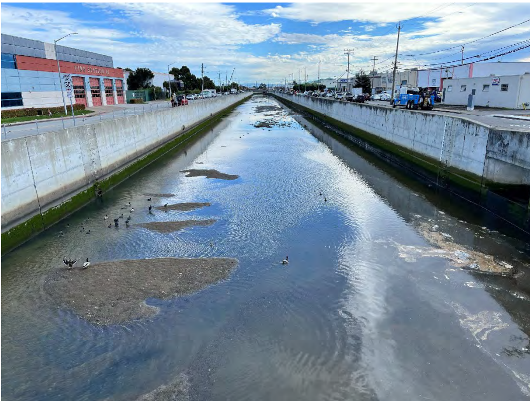
Photos 21 & 22 — Top photo shows Colma Creek looking upstream from Spruce Avenue Bridge. Bottom Photo shows Colma Creek looking downstream from Spruce Avenue Bridge. Low Tide.
