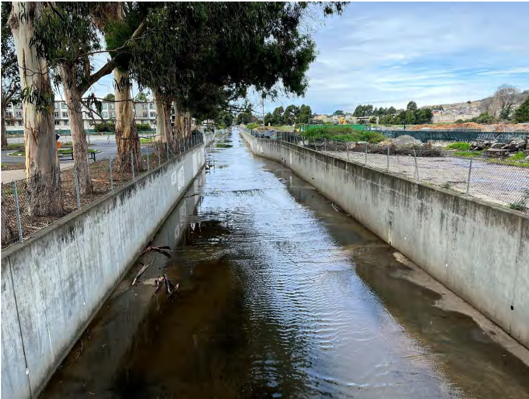
Photos 24 & 25 – Top photo shows Colma Creek looking downstream of the pedestrian bridge in Orange Memorial Park. Bottom photo shows Colma Creek looking upstream toward the 12-Mile Creek confluence.
