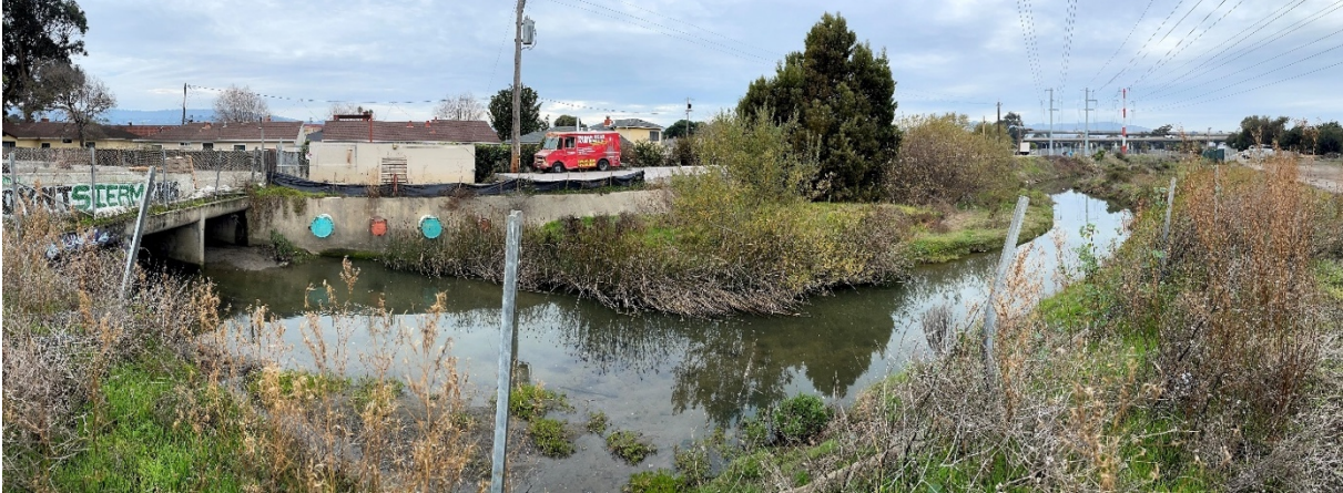
North Channel at Walnut Pump Station
