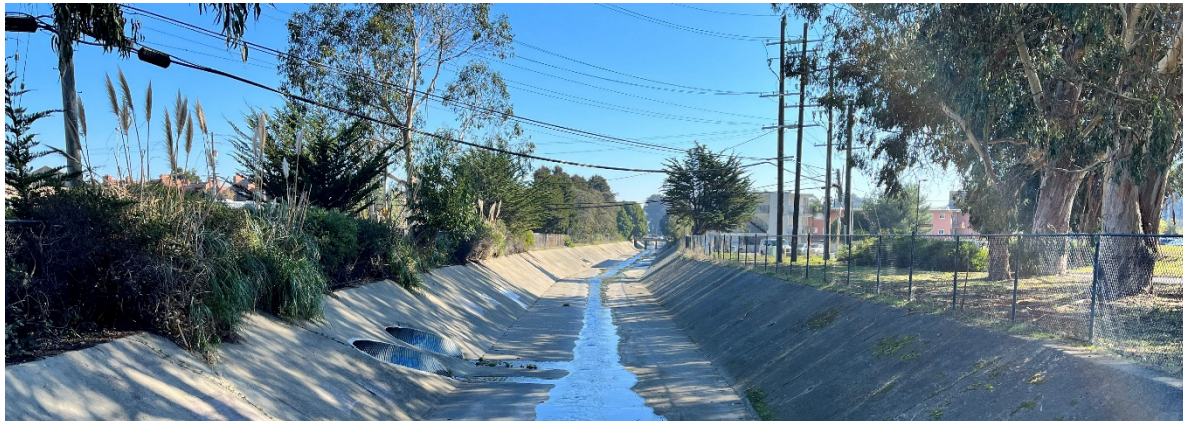
Downstream of Centennial Way
