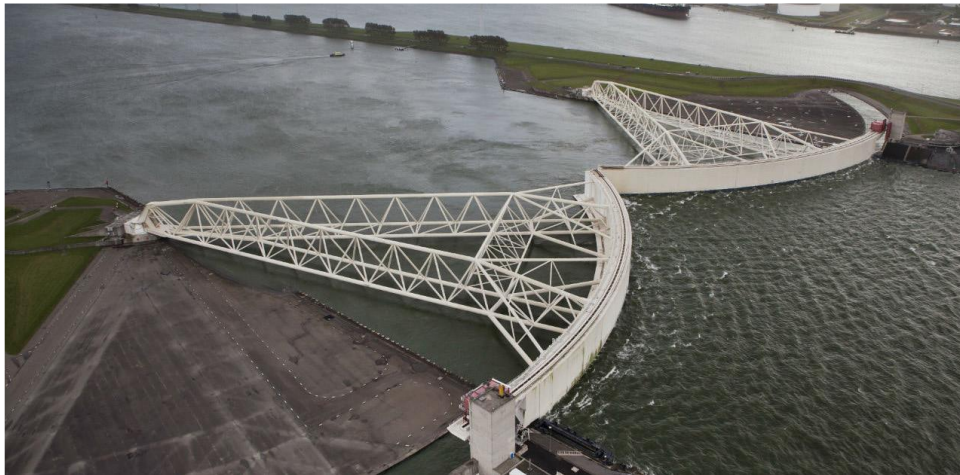
Maeslant Tidal Barrier, Netherlands
