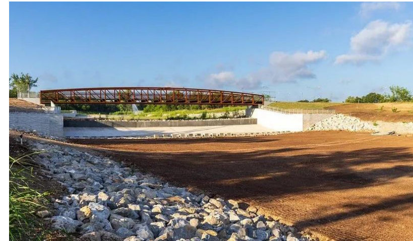
Channel widening at pinch points may relieve existing constraints on water flow, reducing areas of flood risk.
