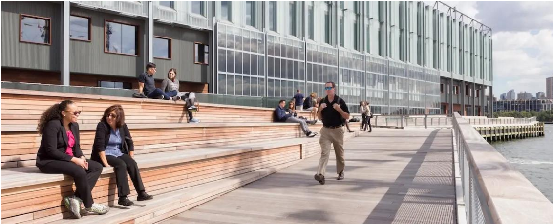
Example: Flood-proofed building, Brooklyn, NY
