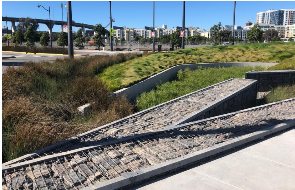
Roundabout Rain Garden
