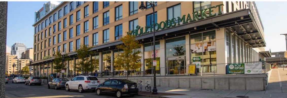
Flood-proofed building, Boston
