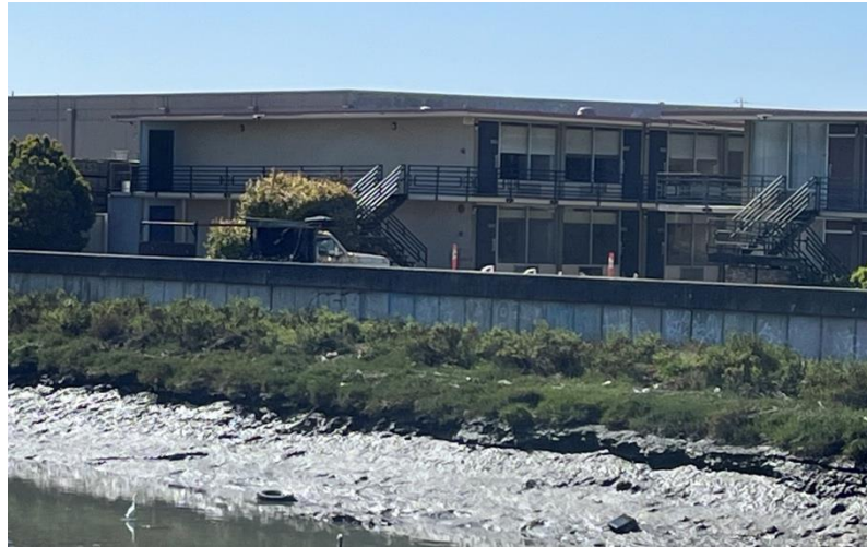
Floodwalls downstream of South Airport Blvd
