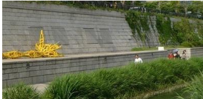
Floodwall with planting and public access
