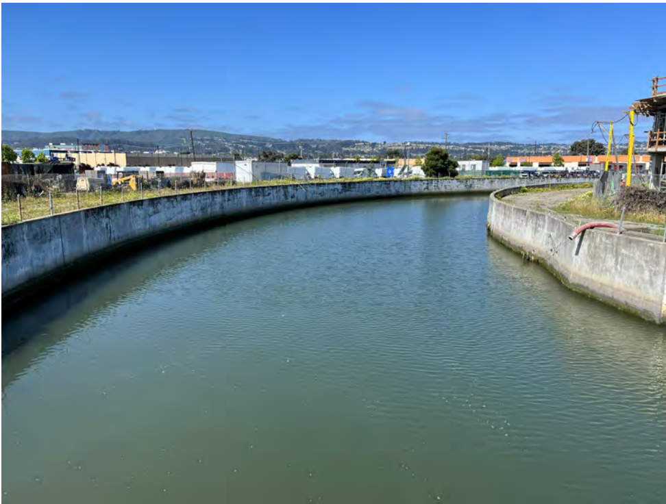
Photos 13 & 14 — Top photo shows Colma Creek looking downstream from the Produce Avenue Bridge facing the US 101 crossing. Bottom photo shows Colma Creek looking upstream from the Produce Avenue bridge. High tide.
