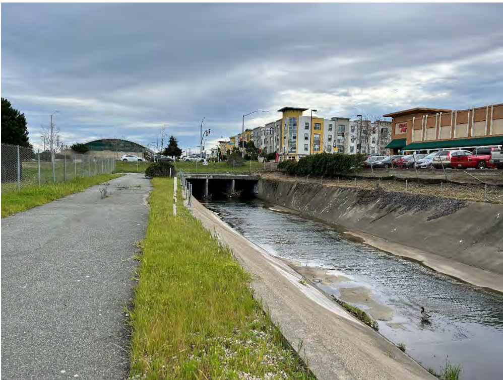
Photos 32 & 33 — Top photo shows Colma Creek looking downstream toward the Old Colma Creek Confluence. Bottom photo shows Colma Creek looking downstream near the Costco pedestrian bridge toward the box culvert.
