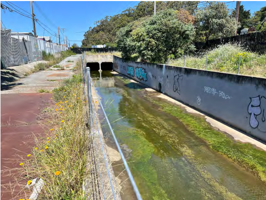
Photos 34 & 35 — Top and bottom photos show Colma Creek looking upstream toward the Mission Road Box Culvert.
